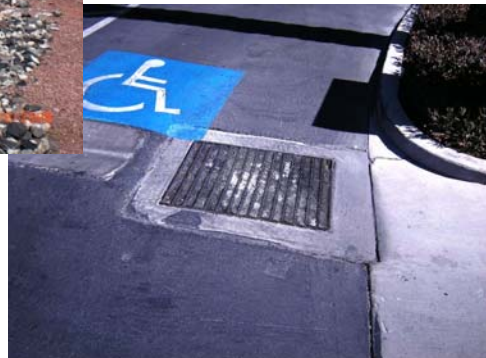
Sediment Deposit at Points of Flow Interception
